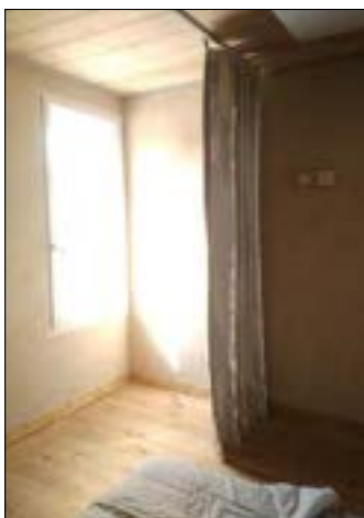
Figure 1.31: A curtain to temporarily create a buffer zone in the SDE19 PLF house. Source: University of Wuppertal, Karsten Voss
