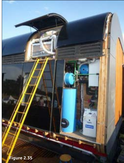
Figure 2.35: Service room with heat pump and thermal storage in an SDE house in 2010 in Madrid.
