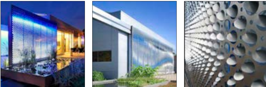
Figure 3.19: Lumen Haus. SDE10. Articulates the architectural space differently through combinations of sliding panels.
