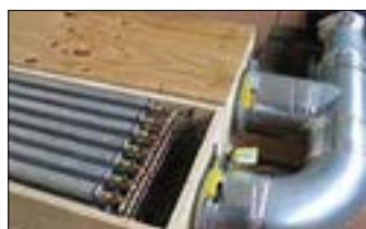
Figure 3.33: Phase Change Material based air tempering system.
