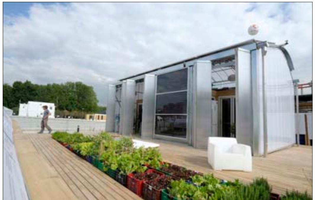
Figure 1.32: A meeting house for a local district with a translucent façade at the SDE10 UPC house. The construction is based on typical greenhouse elements such as multilayer polycarbonate plates. Source: SDE, Flickr [sde flickr doc]
