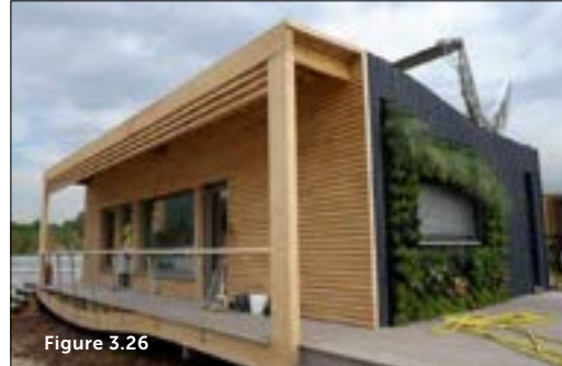
Figure 3.26: Napevomo House. SDE10. Innovative electricity domestic hot water (DHW) co-generation systems.
