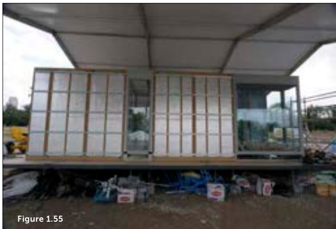
Figure 1.55: Vacuum insulating panels visible at the 2010 UDS (Solarkit) house during assembly.
