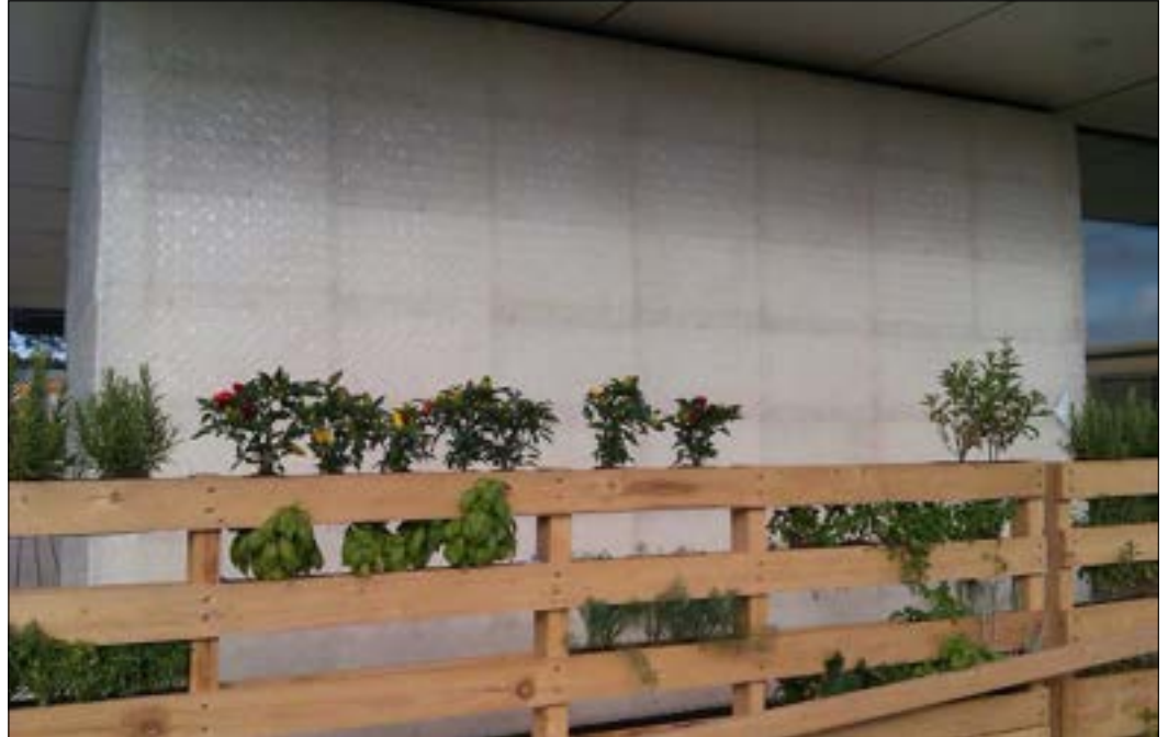
Figure 1.57: Recycled CDs as external cladding at the 2012 RWT house. Source: University of Wuppertal, Karsten Voss
