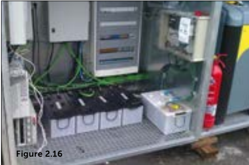
Figure 2.16: Four externally mounted batteries (bottom) with lead-acid technology at an SD house at SDE12. Source: K. Voss, University of Wuppertal
