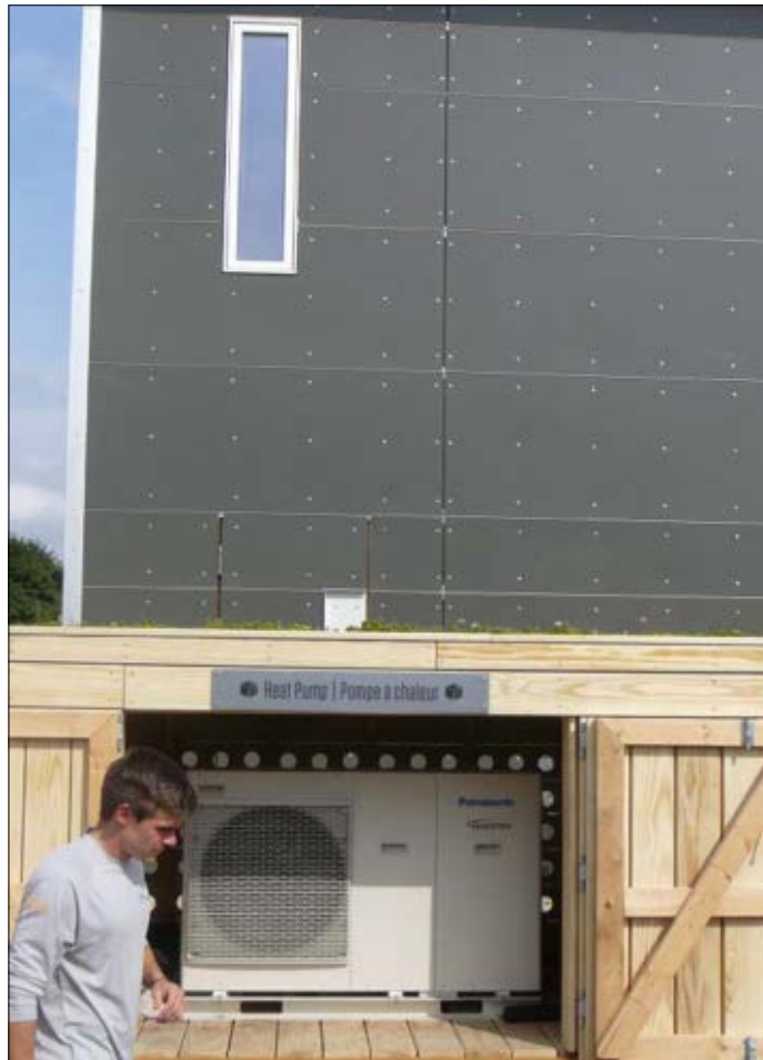
Figure 2.33: Split system compressor outside a building at SDE14.
