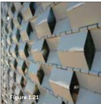
Figure 1.21: Moveable aluminum sun screen at the SDE10 ROS house. The profiles are specially folded to avoid direct light transmittance. The system as a whole is moveable from the bottom to the top and stored at the bottom of the façade. Source: University of Wuppertal, Karsten Voss
