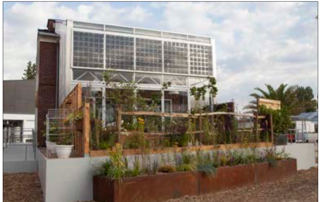
Figure 1.28: The attached conservatory at the 2014 DEL house with integrated solar systems demonstrates a buffer zone example for building renovation.
